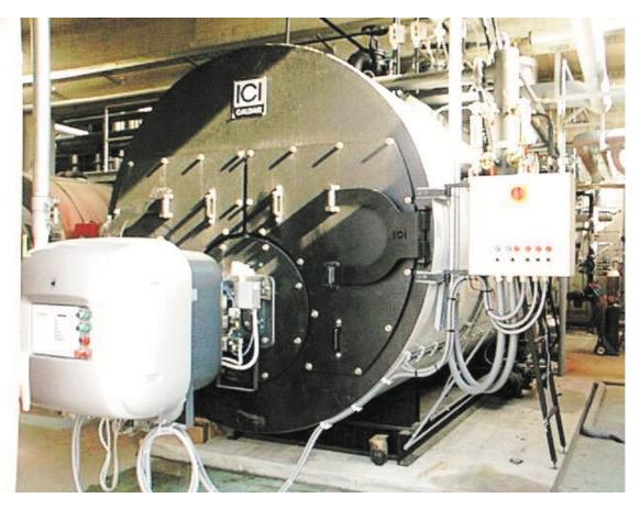
Burner type Burner output Number of units Activity sector Country Installation date MB6SE 5400 [kW] 1 Medical center Italy February 1999 Customer Application Fuel type (....) Boiler make Boiler type Emissions class Note
