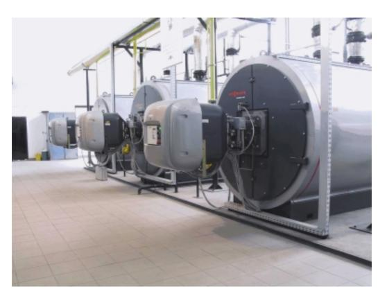
Burner type Burner output Number of units Activity sector Country Installation date MB4SE BLU 3000 [kW] 3 District heating Hungary October 2001 Customer Application Fuel type (....) Boiler make Boiler type Emissions class Note
